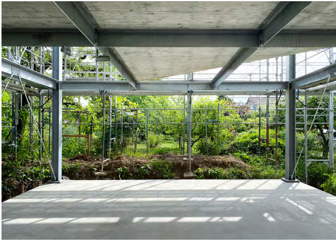
figura 3 Filter House, gentileza COMTE/MEUWLY
