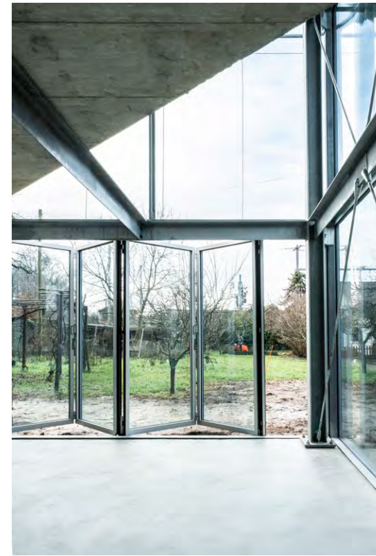
figura 4 Filter House, gentileza COMTE/MEUWLY
