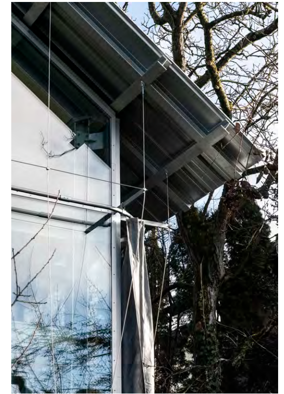
figura 5 Filter House, gentileza COMTE/MEUWLY
